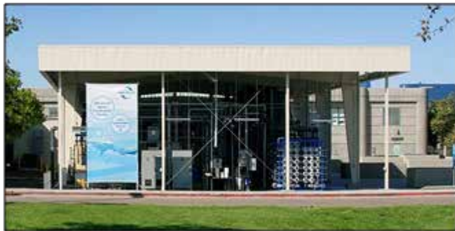
Advanced Water Purification Pilot Plant
